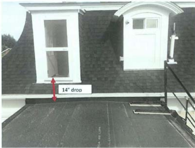
Figure 1. 34 Spring St. Unit 4, egress door, 14" drop to roof level
